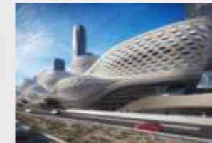
Riyadh Metro, KSA
